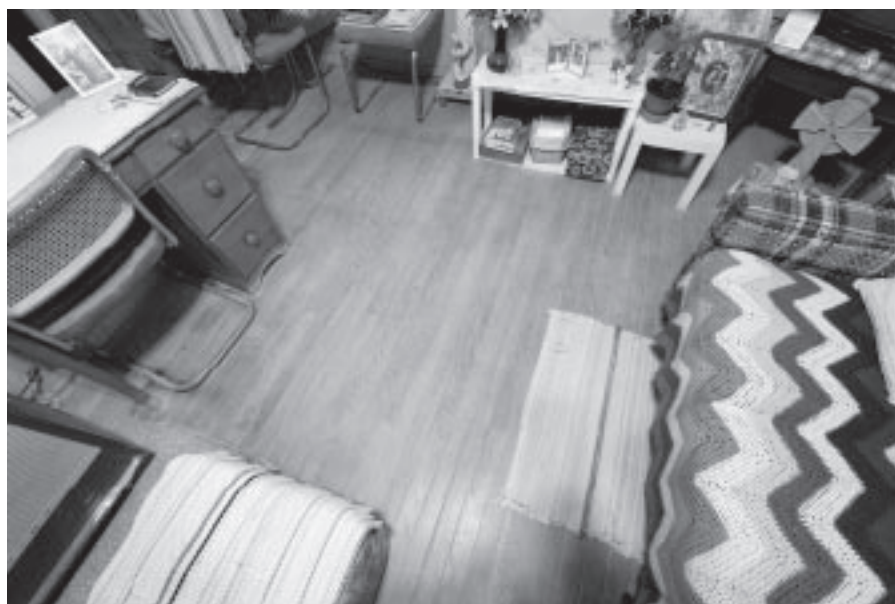
Fig. 25: Hardwood floors, such as this one, were considered inexpensive building materials when installed in 1943. Today they can be harvested for reuse.
