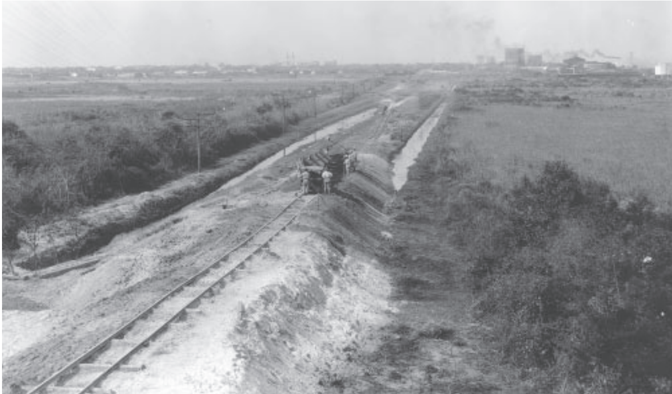
Fig. 7: In 1933, the Deptford Tract remained largely undeveloped. In the view looking westward towards the city, convict laborers work to raise the rail bed.
